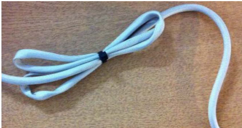
Figure 84 - Securing of excess cable with a cable tie
